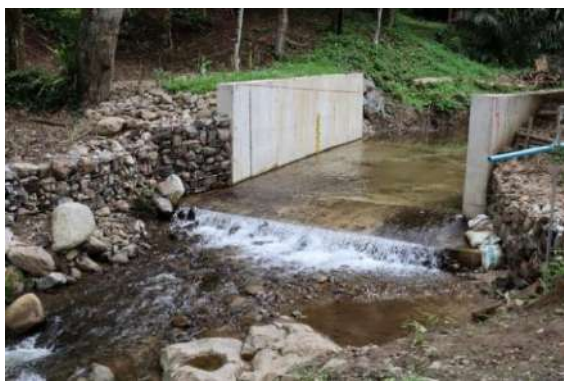
(G) Water Level and Quantity Monitoring Station at the Watershed Management Unit of Khun Kong
