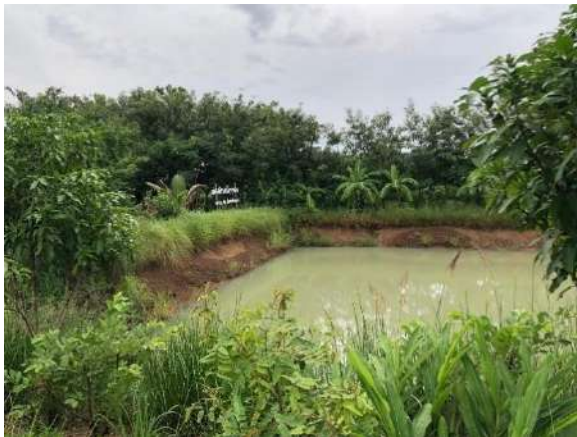
(A) A pond with the planting of vetiver grass to prevent soil erosion
