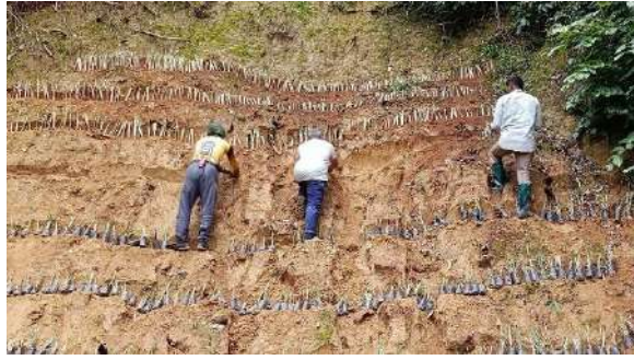
(B) Planting Vetiver Grass to Prevent Soil Erosion in Watershed Areas *
