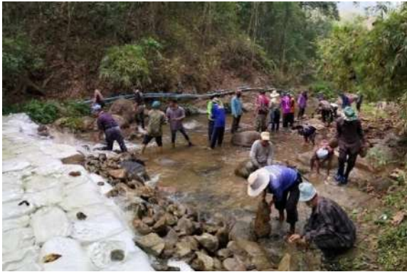
(C) Constructing Check Dams **
